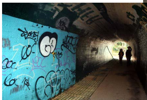
Through the tunnel in the retarding basin dam on Darling Mills Creek. The scheme is designed to prevent the creek from flooding Parramatta in the event of exceptionally rainy times.
